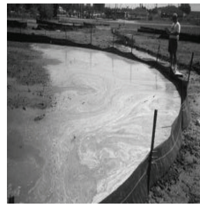
Properly installed silt fence
