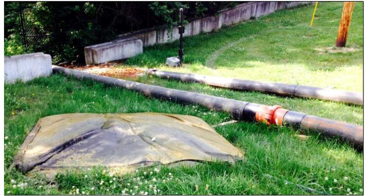
Water from dewatering operations must be filtered before release/discharge offsite. When using a dewatering filter bag, place bag on flat stable surface.
