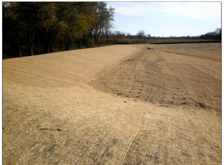
Use the type of Erosion Control Blanket specified in the SWPPP. Prepare the area by removing rocks or clods over 1-1/2" in diameter. Anchor blankets in place.
