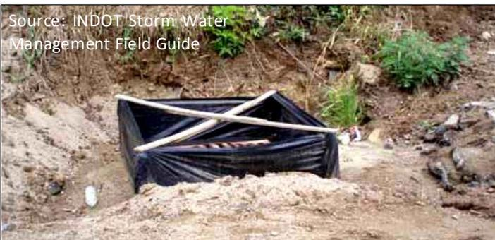
There are multiple options for inlet protection: geotextile box with cross bracing; gravel ring (riprap with 12" of filter stone); commercial inlet filter products.
