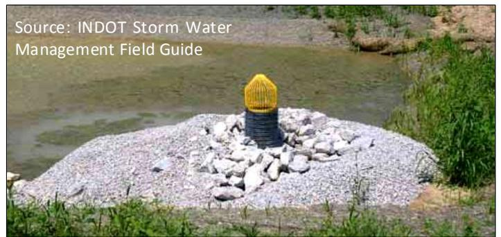
Install per SWPPP specifications. Clear/grub/prepare sub-base. Install Principal Spillway. Install embankment for pool area. Install emergency spillway.
