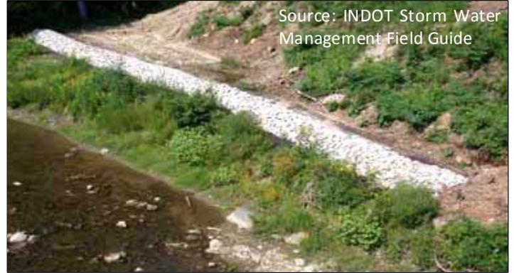
Filter berms can be made of rock, compost or filter sock. When using rock, place riprap on geotextile fabric with filter stone (#5 or #8) on the upslope side.
