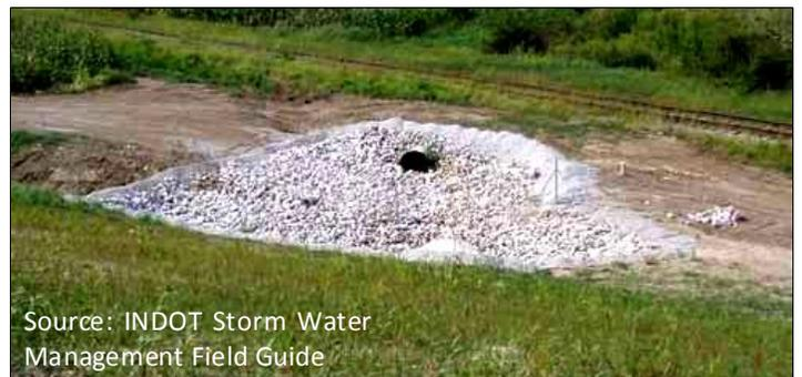
Install culvert inlet protection as identified by the SWPPP. Place revetment riprap to create the basin at the culvert. Place #5 or #8 stone as a filter around the perimeter.
