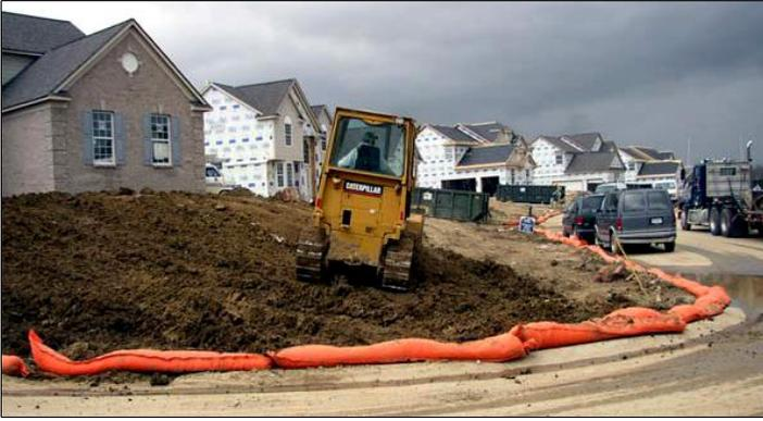
Place filter sock barrier at least 10 feet past the toe of the slope and place filter sock to be parallel to the slope contour. Overlap ends of filter sock.
