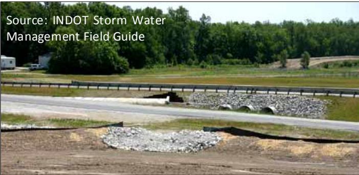
Install at location as identified by the SWPPP. Place geotextile fabric and revetment riprap. Line inside face with 12" layer of #5 or #8 stone. Stabilize outlet.
