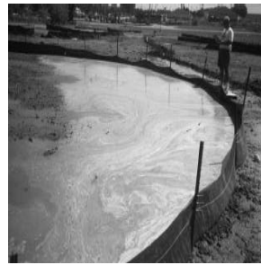
Properly installed silt fence
